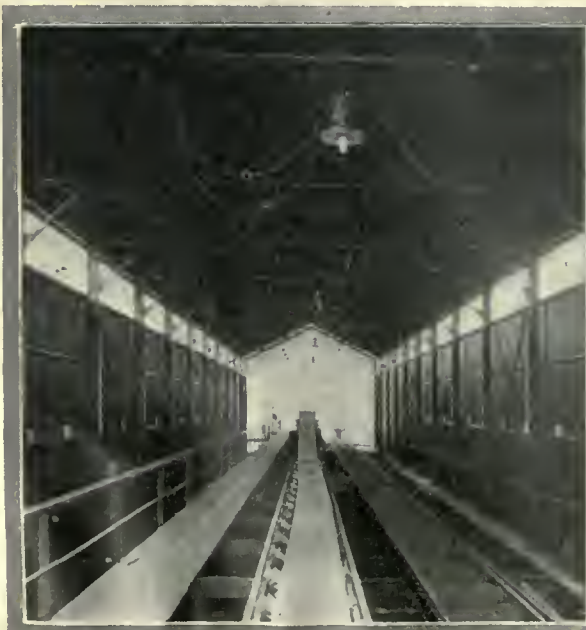
UPPER FLOOR OF FEED-BIN BUILDING.
